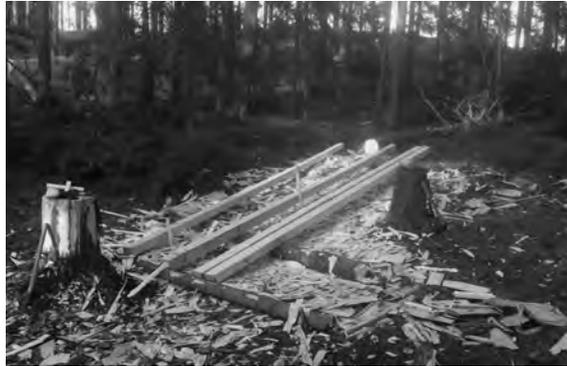
*Fig. 7 During the season 2014 we made an experiment with producing four 7 metres long rafters from one log. The boxing and the cleaving was done where the tree was felled. The rafters can be seen in between the stump and the top of the tree. The waste was minimal. Photo Karl-Magnus Melin.*
