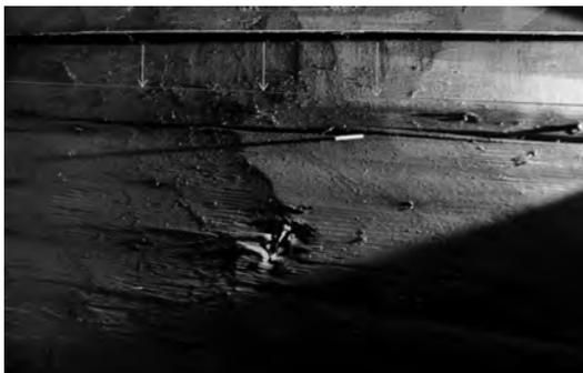
Fig. 2 Traces of *spårning*. The arrows show the direction the axe was driven down plumb. Photo Daniel Eriksson.
