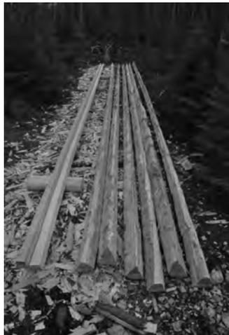
*Fig. 8 From one log we could produce eight 13 metres long rafters. The two rafters to the left are completed. We carried out the completed rafters with no problem. Photo Daniel Eriksson.*
